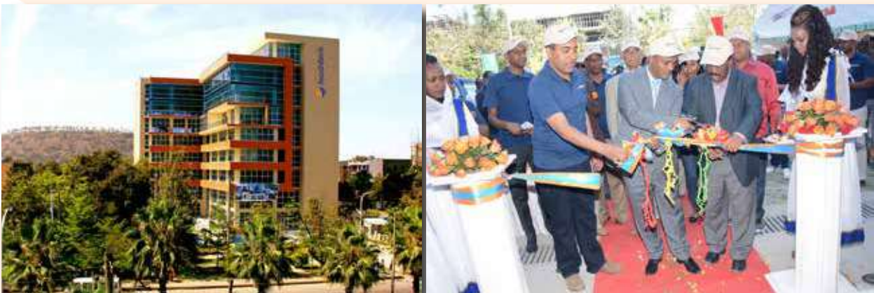
Inauguration Ceremony of Awash Bank's Hawassa Building in the presence of H.E. Meles Alemu, V/President, SNNP National Regional State and Head of Urban Housing & Development Bureau
