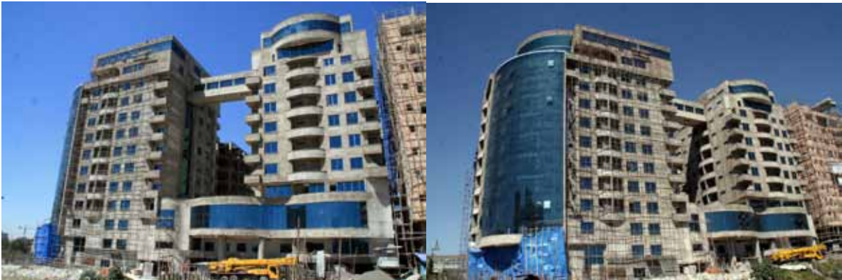
Hotel under construction: Kazanchis, Addis Ababa
